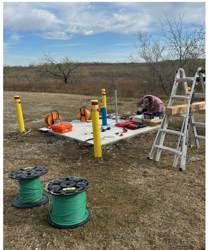
Field Technician, Jose Sarmiento, installs equipment on newly drilled monitor well.
