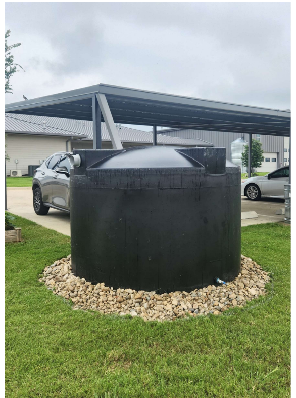
The District installed a new rainwater harvesting system with three 1,500 gallon poly tanks.
